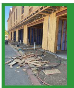
Poor housekeeping around the buildings lose lumber on the floor with some nails sticking up. Please nail down all nails that are sticking up. Housekeeping- §1513. Housekeeping. (a) During the course of construction, alteration, or repairs, form and scrap lumber with protruding nails and all other debris shall be kept reasonably cleared from work areas, passageways, and stairs in and around buildings or other structures.
