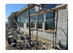
Missing cross brace for front side of scaffolding
