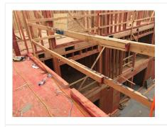
Guardrails exceed 8' between vertical posts.
