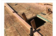
An access ladder to the top floor is not protected by a corral.
