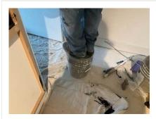
An employee is standing a bucket to gain elevation, which is not permitted. Please ensure employees use approved means of gaining elevation, such as a ladder.
