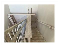
Scaffold planks are setup on ladders and stairs as an unapproved makeshift scaffold. Please ensure approved materials are used to setup scaffolding under the direction of a competent person.
