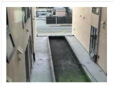
A top rail is missing where required on the podium level. Please ensure railing is installed at 42-45" top rail, with a. Mid rail halfway between the top rail and the working platform.
