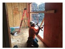
An employee has removed the guardrails that were installed in order to complete his task. This exposes the employee to a significant fall hazard. Please ensure the employee implements personal fall protection.
