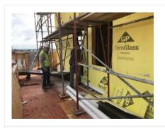
Employees have removed guardrails to move materials into an elevator shaft. This exposes them to a significant fall hazard. The employees must implement a means of fall protection, which likely will be through the use of personal fall protection.
