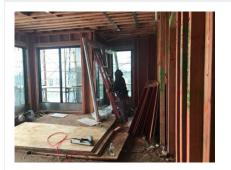
An employee was using an A-frame ladder in a closed position. Please ensure employees use their ladder in an open, locked and level position, which may require housekeeping prior to performing the task.
