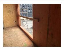
A mid rail has been removed where required. Please ensure a mid rail is installed halfway between the top rail and the working platform.
