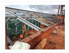
Guardrails have not been installed where required. Please ensure guardrails are installed at 42-45" top rail, with a mid rail halfway between the top rail and the working platform.
