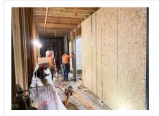
Employees are working at the opening of an elevator shaft while not using personal fall protection. This exposes them to a significant fall hazard. Please ensure fall protection is implemented.
