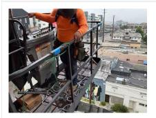
An employee using a boom lift does not have his leg straps secured, his harness is looped around itself and to a guardrail, and he has an excessive amount of slack in his lanyard.
