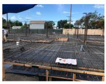
Pictured is rebar that has not been capped or covered.
