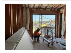
Employees are stocking drywall and have removed guardrails, which exposes them to a significant fall hazard. Please ensure a means of fall protection is implemented.
