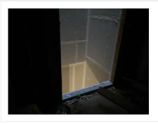
A floor opening has been left open without guardrails installed, which exposes a significant fall hazard. Please ensure guardrails are installed.
