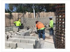
Employee is not maintaining sufficient water to control the dust while cutting block.
