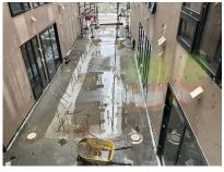
Rebar has not been capped, covered, or bent down. Please ensure impalement protection is provided.
