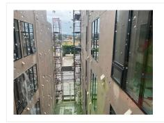
Missing guardrails were observed on the scaffold. Please ensure guardrails are installed where required.
