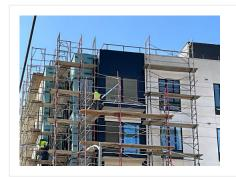
An employee was observed climbing from the balcony onto the scaffold, which due to the distance is not permitted. Additionally, end rails are missing in a section of scaffolding.
