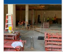
Caps are needed for this rebar as it is an impalement hazard.
