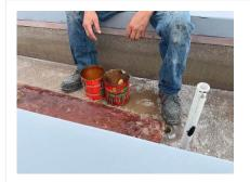
Employees are applying resin to fiberglass in an enclosed area, which creates an inhalation hazard. Although the employees are in the roof, their location likely requires them to use a half mask respirator.
