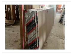
Drywall that is leaned against a wall must be secured from tipping, slipping, and falling.
