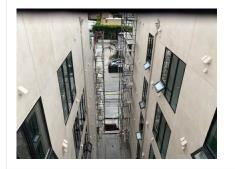
Missing guardrails were observed on the scaffold. Please ensure guardrails are installed where required.
