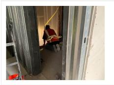
An employee is exposed to a fall hazard while working on an unprotected edge. Please ensure a means of fall protected is implemented.
