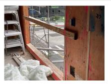
A missing guardrail exposed a fall hazard on the 3rd floor. Please ensure railing is installed.
