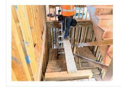
An employee is using a single plank on a ladder as a means to gain elevation, which is prohibited. Please ensure the employee uses an approved means of gaining elevation, such as scaffolding.
