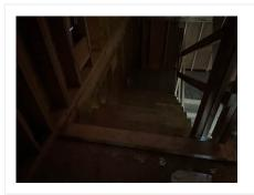
Illumination is lacking in a section of stairs. Please ensure lighting is provided.
