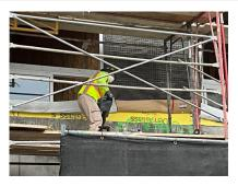
An employee is chipping concrete while not using engineering controls, such as a continuous water supply or a HEPA vac. Please ensure engineering controls are present, used, and maintained.
