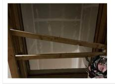
A guardrail appears to have been lowered and not reinstalled at the required height. Please ensure the top rail is installed,led at 42-45" height.
