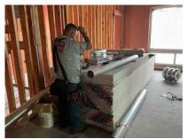
An employee was observed cutting an aluminum pipe with a grinder while not wearing a face shield. Please ensure employees are wearing the proper PPE.
