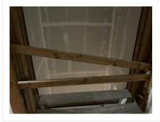
A guardrail appears to have been lowered and not reinstalled at the required height. Please ensure that the top rail is installed at 42-45" in height.
