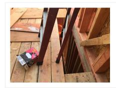
Opening is not fully covered, which creates a fall hazard.
