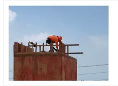
Employee is using a nail gun while not wearing safety glasses. Additionally the employee is not wearing a hard hat, which is required while on the jobsite.
