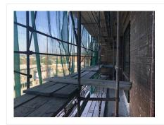
Scaffolding is missing guardrails where the planks exceed 16" from the structure.
