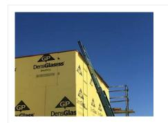
Ladder does not extend 36" above the platform being accessed and it is not secured from tipping.
