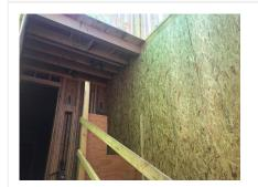
Stairs have not been provided for access to the top floor, which creates a hazard in the event of an emergency.
