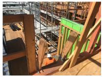
This access ladder does not have a corral or removeable guardrail installed.
