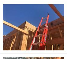
This access ladder has not been secured from tipping, slipping, or falling.
