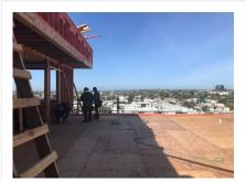
Employees are working above their trigger height while inadequate railing is provided. The scaffold does not have the required guardrails installed and the top tie anchor is not secured within a 3:1 height to width ratio from the top of the scaffold.
