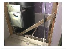
A trash chute was installed yesterday. Existing railing was removed, creating a fall hazard.
