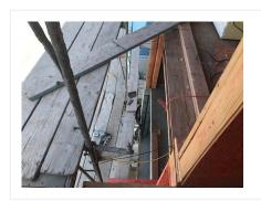
Proffer employees are using a section of scaffolding that is missing the required planks and railing.
