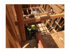
Framer is using the top steps to transfer from the upper platform to the lower platform.
