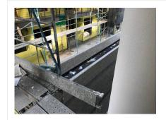
Guardrails are missing in the pictured area, which exposes a significant fall hazard.
