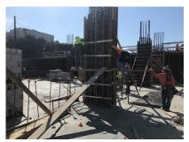
Employees are using a single plank for scaffolding, which is unapproved.
