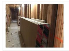
Drywall that is leaned against a wall has not been secured from tipping, slipping, or falling.
