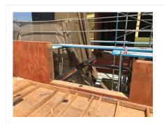
Railing is lacking in a section where scaffolding exceeds 16" from the structure.
