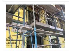
A section of scaffolding is missing the required planks.
