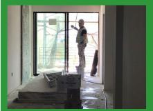
An employee is using a bucket as a means to gain elevation, which is prohibited.
