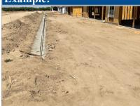
CVC Concrete missing rebar caps on rebar.
