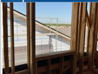
McDaniel Construction framers missing top guardrail on second story window opening. **Example:**
