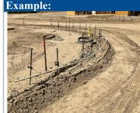
CVC Concrete missing rebar caps on rebar.
