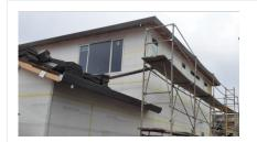
found a section without the proper railing/fall protection from scaffolding to the roof
