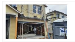
scaffolding does not have a ladder or the correct about of planks in the correct location
