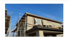
need guard rails in place from transition from scaffolding to the roof
