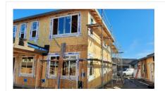
I found scaffolding that does not have proper guard rails in multiple areas, a unfinished section and no ladder
