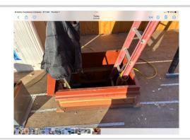
Are extension ladders in safe condition, set up at a 4:1 pitch, secured, and extend at lest 3' above the roof platform?
