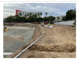
This sloped wall needs to be benched, and sloped according to the soil type. Also, it is not recommended to put heavy items at the top of the sloped wall.
