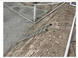
Workers cannot use an A Frame ladders to exit the excavation
