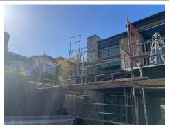
Toe board is in place on upper level in this photo where stone is present on the scaffolding. Toe board is needed on lower level also.
