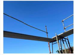
Midrail is missing and adjoining midrail is unattached to frame.
