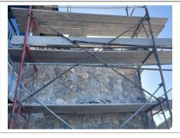
Plank is missing. All frames must be fully planked.
