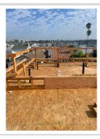
Window opening on second floor requires a guardrail as it is less than 36" off the floor with a drop of more than 4 feet. Corrected on the spot.
