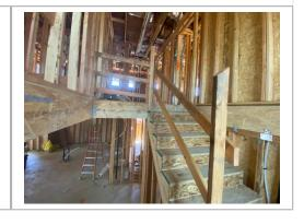
Rail is loose at the bottom section of the stairs. The bottom post needs to be secured.
