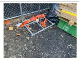
Installed support is a hazard. Ensure that it is protected.
