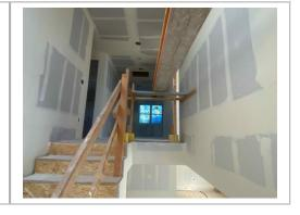
Makeshift platform added to the top of the stairwell. This is a greater than 7 1/2 feet fall hazard. This is not allowed. It is unclear which subcontractor put this year because it was not being used and no one was working on the interior of the house at the time. However, it is suspected this is that this is related to drywall finishing.
