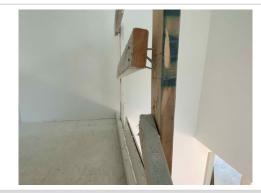
Additional photo of guard rail installed incorrectly.
