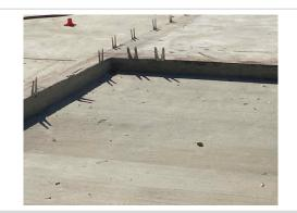
Nail sticking out of the foundation or a hazard. Ensure they are bent over or cut off.
