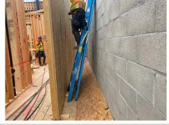
One more Trademark employee is using an A-Frame ladder in a closed position. Please ensure employees use ladders in an open, locked, and level position. Alternatively, a lean-safe ladder may be used.
