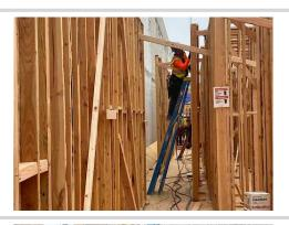
Another Trademark employee is using an A-Frame ladder in a closed position. Please ensure employees use ladders in an open, locked, and level position. Alternatively, a lean-safe ladder may be used.
