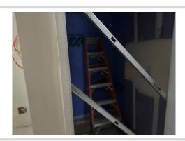
Shaft protection has been removed and left loose. The shaft must be protected at all times.
