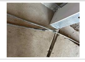
Rye has an electrical cord with damaged insulation. The cord must be removed and replaced. The workers complied to remove the cord immediately.
