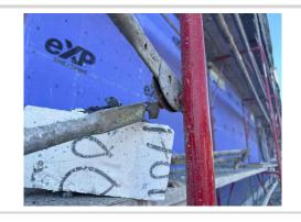
Guy Yocom scaffold in stairwell is missing planks with open gaps to the level below. Please ensure all working levels are fully planked.
