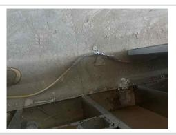
There are several bulbs missing from light strings. Light strings must be inspected regularly to ensure all bulbs or manufactured caps are in place to eliminate any shock exposures.
