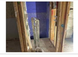
Please ensure all window openings on the mezzanine level are protected with guard rails. This opening is unprotected.
