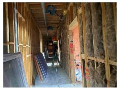
Trademark worker has a leaned A Frame ladder. Please ensure the ladder opened and locked when in use. A LeanSafe ladder may be used in this application.
