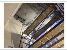
Sharp has a plank on top of a self supported ladder to a the top of a guard rail. This is prohibited. Planks may not be extended from ladders. Please ensure proper scaffold frames are used as well as the minimum width of 20" for a scaffold platform is used.
