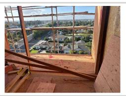
A top guard rail is missing above the trash dump. Please ensure all guard rails are in place at all times.
