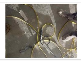
Temporary leeds have been fixed with electrical tape. Please ensure these are replaced as electrical tape is not approved for temporary extensions of power. Ground level near the elevator.
