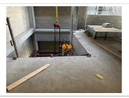
Guy Yocom workers are exposed to fall hazard wiring without guard rails. The work consists of finishing block columns. The guard rails must be in place where workers are exposed and no work is accomplished. The workers complied to erect guard rails immediately.
