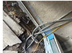
The temporary cord has been damaged. Workers transporting materials must be careful not to damage temporary power extension cords. Near unit 433.
