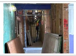
Trademark worker is observed climbing the ladder while holding the nail gun. This is prohibited. Three points of contact must be maintained while ascending and descending the ladder. Reported to his forewoman.
