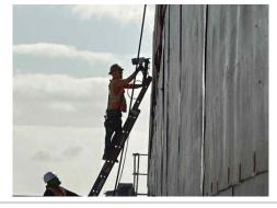
Rye worker is standing on an unleveled A frame ladder. The A frame must be leveled before workers engage it for use. The worker complied to place it on the level floor.
