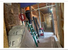
Trademark worker is using the A frame ladder as a leaned. This is prohibited for this ladder. Please ensure all workers are trained regarding proper ladder usage and regulations are followed. The worker complied to open the ladder.
