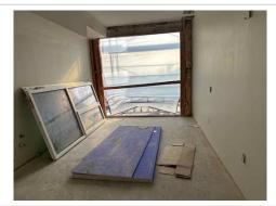
A window opening in 608 is observed with only one rail. Please ensure standard rails are setup at 42/21".
